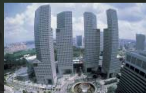
The five office towers are served by dedicated elevators for different floor zones.
