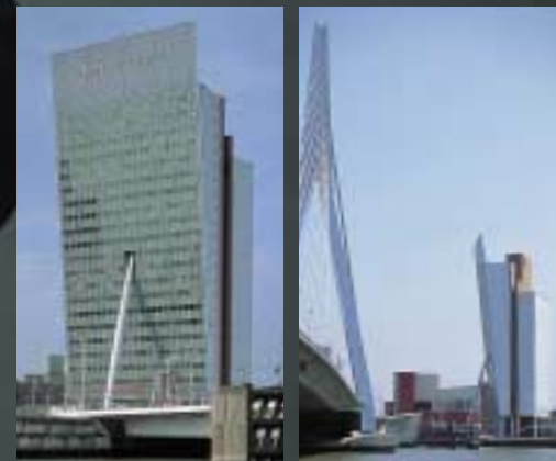
The slanting front wall of the KPN Tower, Rotterdam.
